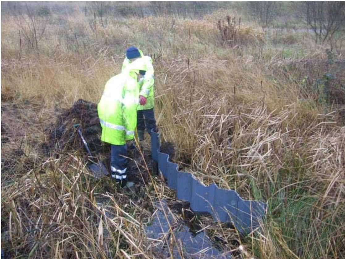
Installing plastic piling dams at Red Moss
